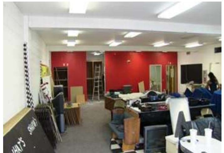
With stuff moved to the middle, remodeling begins for platform.
